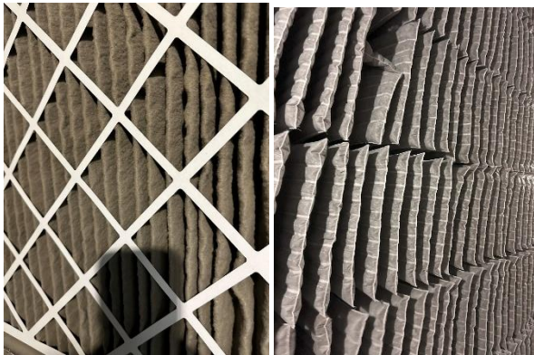
MERV 13 Pleated Filter (left), Bag Filter (Right) of Perimeter Supply Fan
