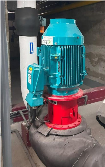
Primary Chilled Water Loop Pump
