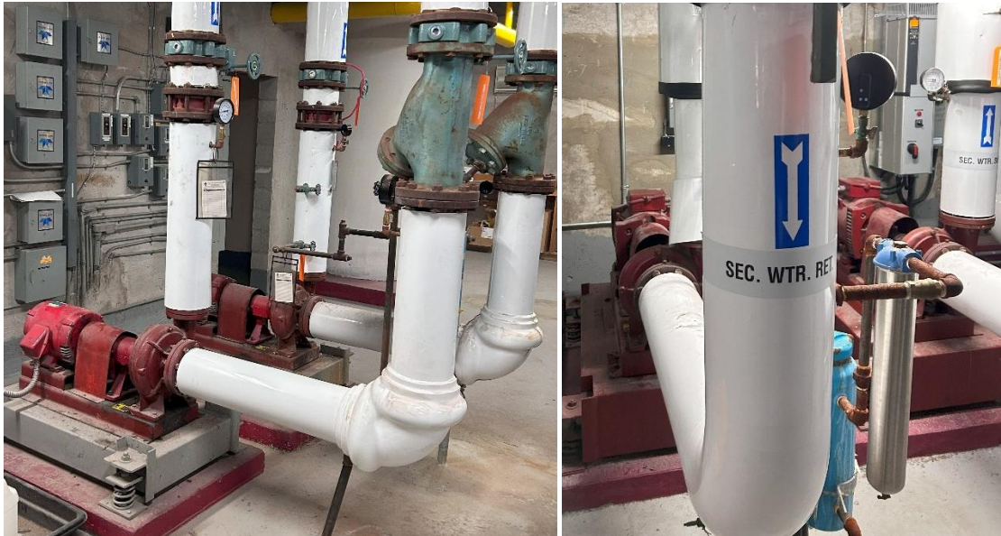
Primary Pumps (left), Secondary Pumps (right)
