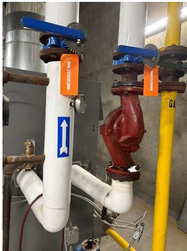
Circulating Pump for Boiler #1
